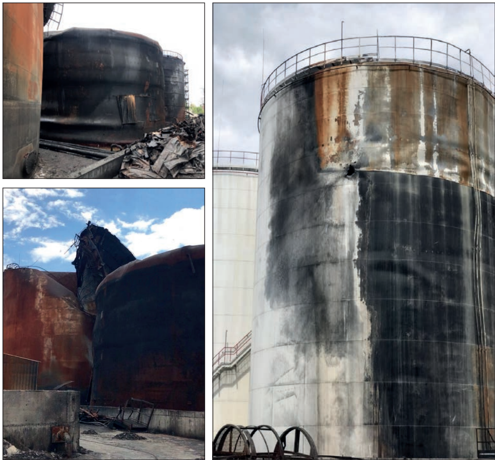
Fig. 5. Consequences of a missile strike on tanks with sunflower oil [32]
